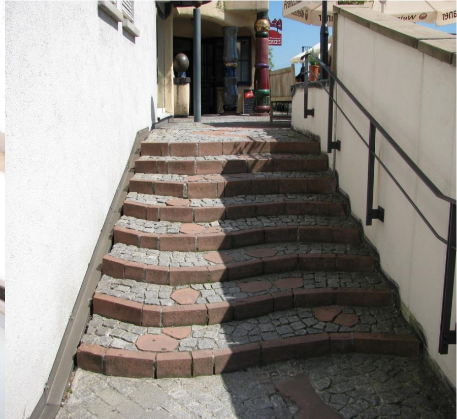
Inaccessible Shopping Area
