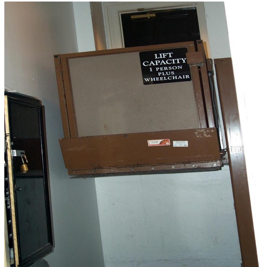
Retrofitting Lift to ADA requirements
