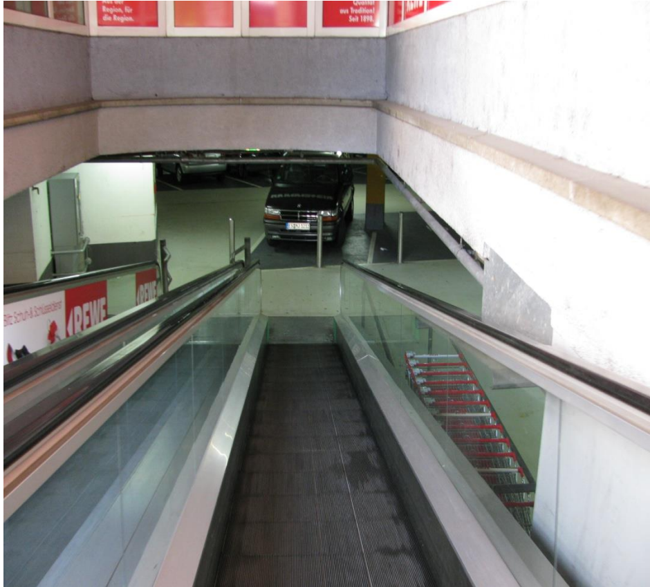
Accessible Moveable ramp from the Garage
