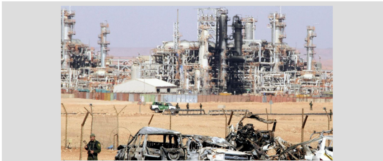
Figure 2: Gas facility, Amenas, Algeria, 16 January 2013.
